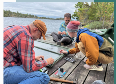
Window work, Carpentry Work Week
