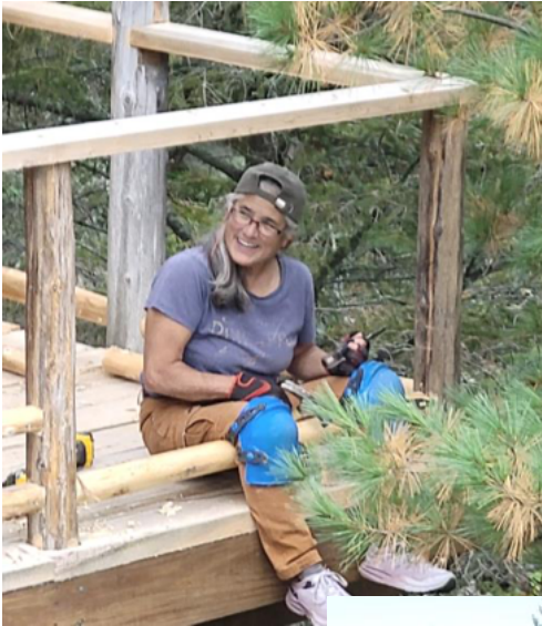
Putting finishing touches on Big House west deck.
