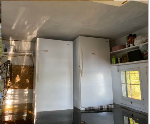
Pump House appliances lifted to the ceiling!
