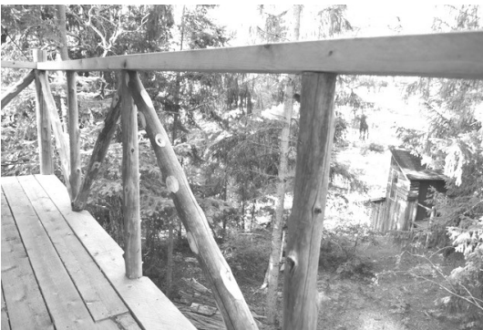
Finished railing on the balcony at Bird House
